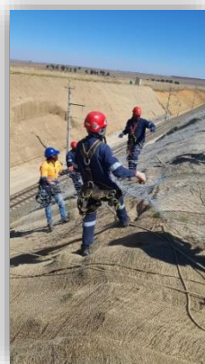
(d) Ensure the HTS mesh is aligned and placed flat along the ground.
