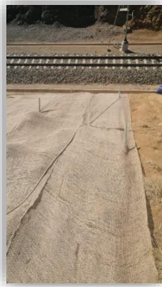
(b) Place natural erosion and growth medium mat.
