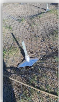
(e) Anchor / Mesh connection is critical. Ensure the transfer of tensile force into the HTS net. Locked / Clamped.
