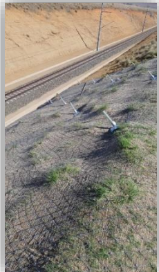
(f) An offset anchor grid pattern, maximizing anchorage support.
